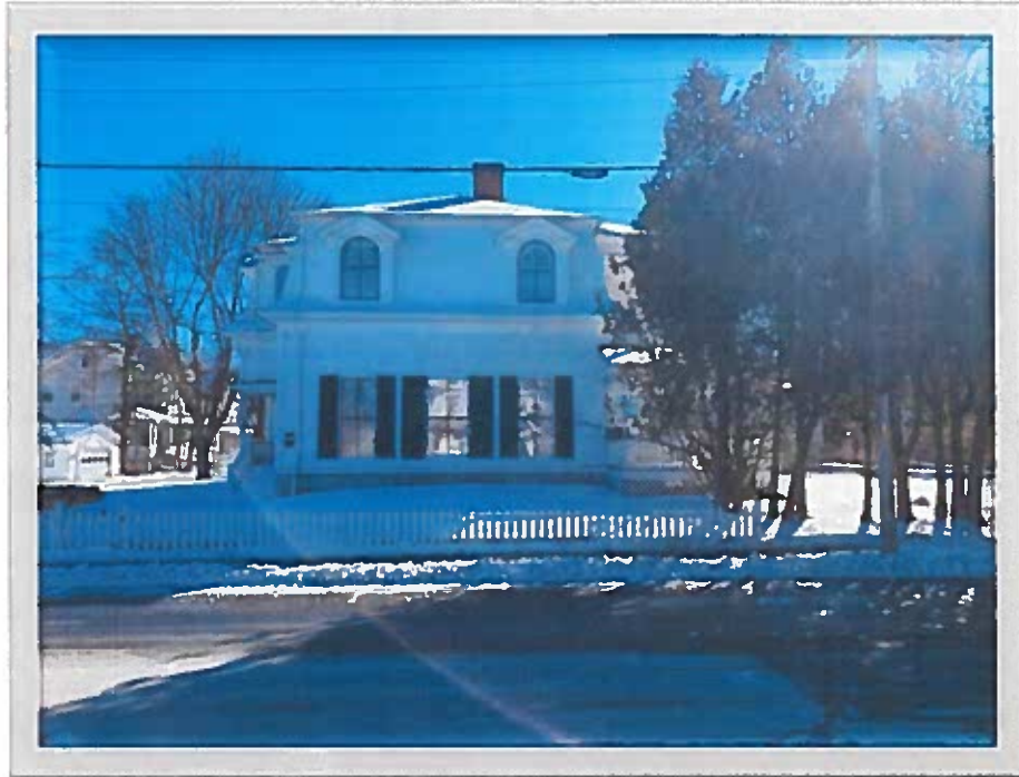
SUBJECT PROPERTY 112 WEST STREET VIEW
