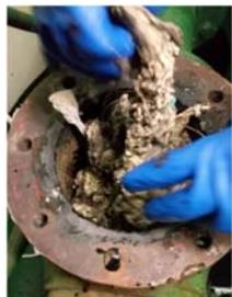
FLUSHABLE WIPES AND FLOSS BEING PULLED FROM EQUIPMENT IN BAR HARBOR
